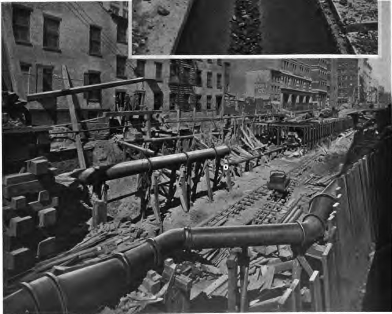
LARGE GAS AND WATER PIPES, RELAID BEHIND EACH SIDE WALL ON ELM STREET
